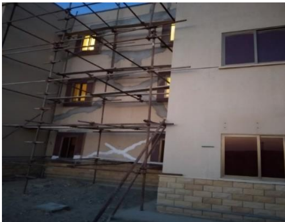
Figure 9. Repaired cracks at PAF base at Bholari
